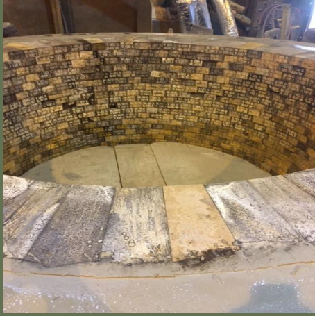
1. MIG Refractory Products Mag Chrome Brick installation (Left Photo)
